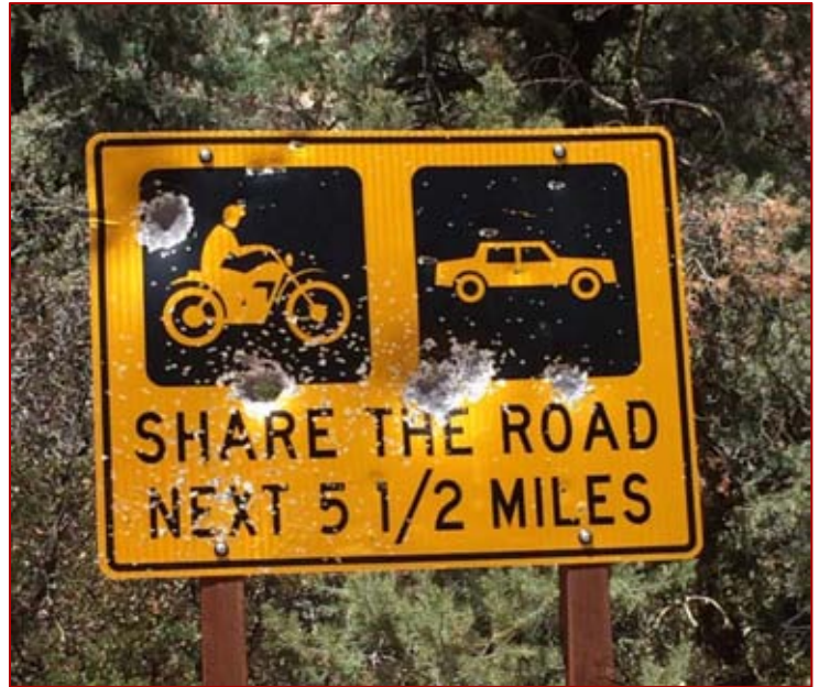
ONE OF MANY DAMAGED SIGNS FOUND THROUGHTOUT THE MPRD
